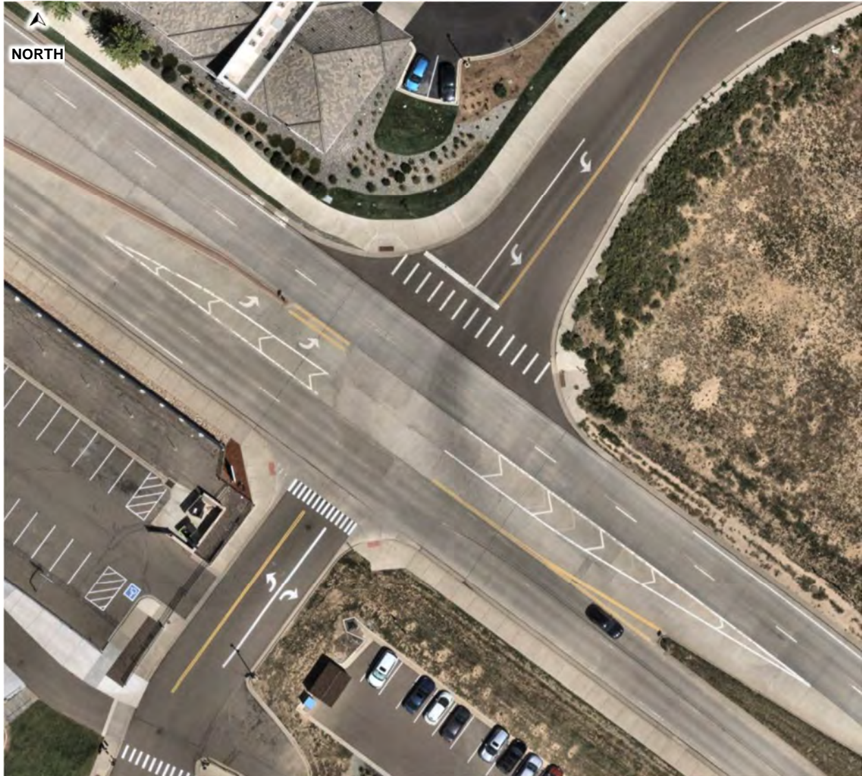
Plaza Circle and Plaza Drive (#2)
