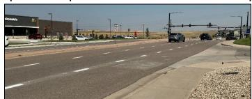
modifications to pavement markings on the eastbound Waterton Road approach to Rampart Range Road. This work included removing existing pavement markings and installing new channelizing markings to extend the right-turn lane. The changes will allow vehicles on Waterton Road to access the right-turn lane from 430 feet upstream
