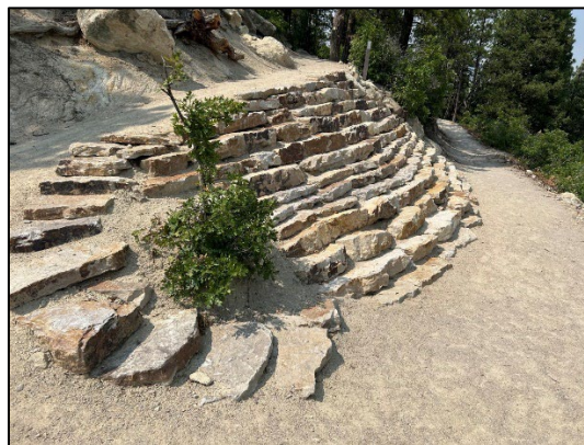
Newly added retain stones on a trail switchback to stabilize erosion and improve drainage
