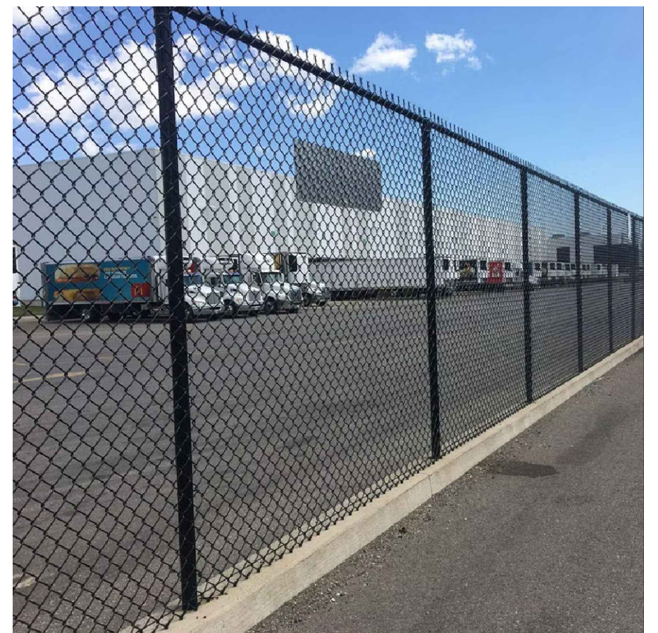
EXAMPLE BLACK PVC CHAINLINK FENCE N.T.S
