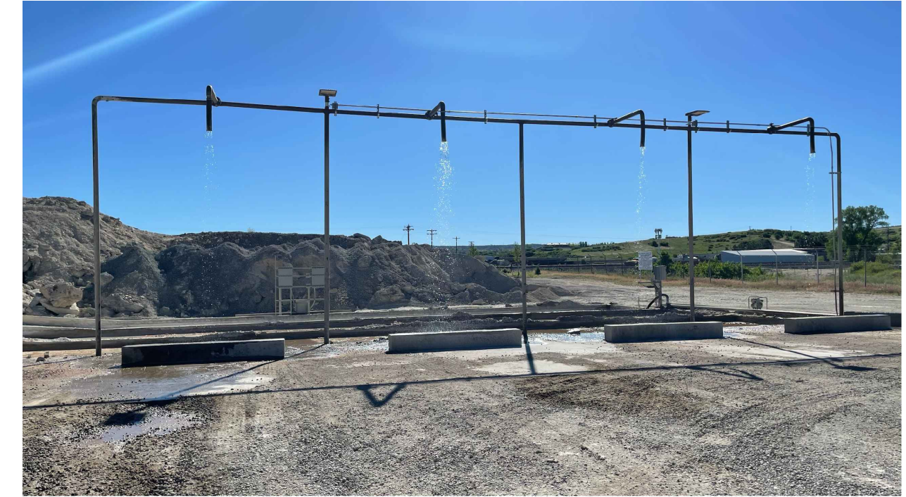
EXISTING TRUCK WASH OUT FACING EAST
