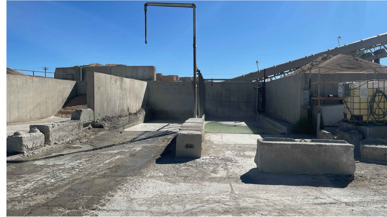
EXISTING TYPICAL MATERIALS BIN AND WASHOUT FACING EAST
