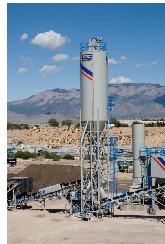
LIME SILO Notes: Painted: Beige Height: 71' - 8" Width: 11' - 11" Length: 11' - 11"
