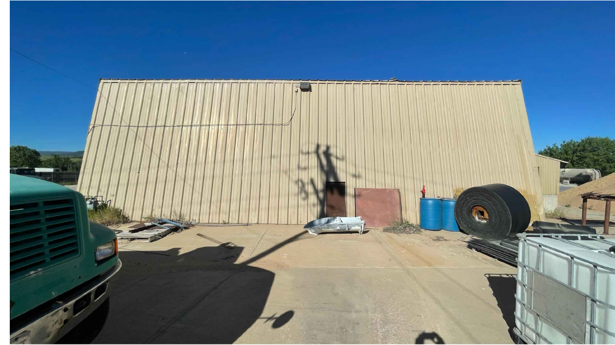
EXISTING MAINTENANCE BUILDING AND OFFICE WEST ELEVATION
