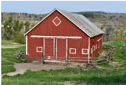
Before project work
