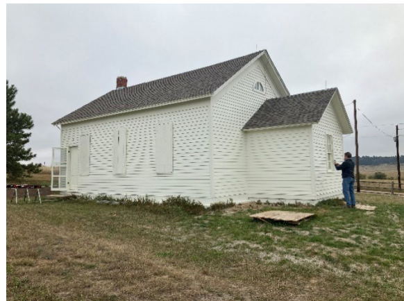
During restoration work
