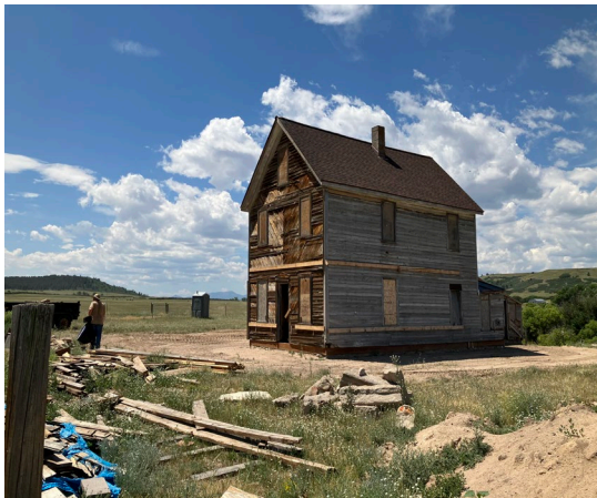
Before Phase 2 Construction
