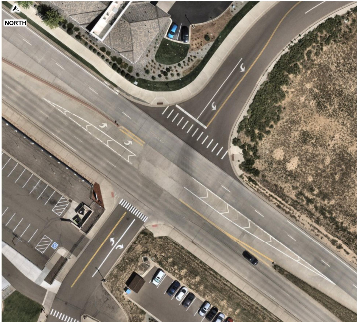
Plaza Circle and Plaza Drive (#2)
