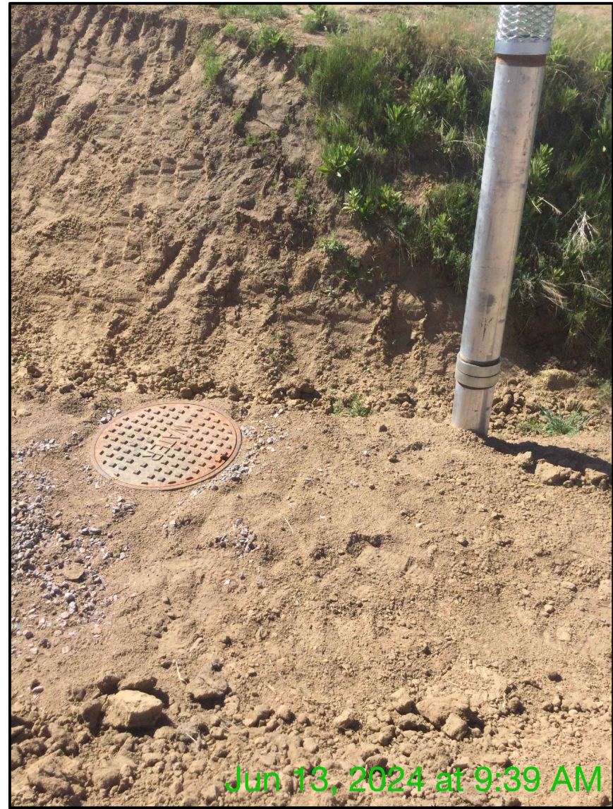
AIR RELEASE VALVE & VENT
