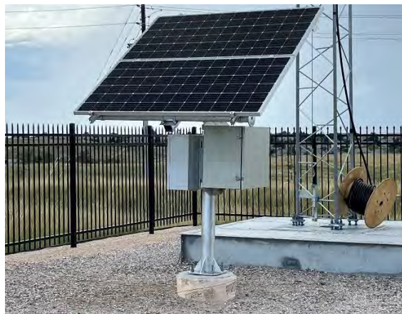
Figure 2: AMI Controls and Solar Panel
