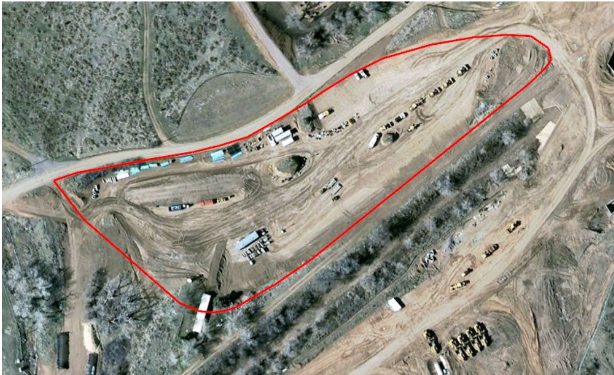
Figure 3. Google Earth imagery from 2006 shows near complete disturbance of the project area. By April 2007, the modern mobile home (southwest) was removed and the remaining surrounding area was disturbed (Google Earth 2024).
