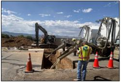
• **Dad Clark Gulch** - Work is underway to mitigate severe erosion along a section of Dad Clark Gulch, just south of Highlands Ranch Parkway. The stabilization improvements include raising and restoring the historic channel elevation, developing a riffle-pool stream patter, and integrating bioengineered bank protection to increase channel stability and vegetation cover.
