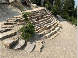
Newly added retain stones on a trail switchback to stabilize erosion and improve drainage
