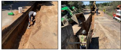
• Bear Ridge Subdivision - Nordstrom Construction is installing a sanitary sewer (DV#2021-287).
