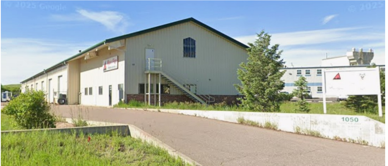
SUBJECT: EXTERIOR OF BUILDING #1
