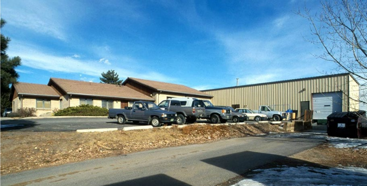
SUBJECT: EXTERIOR OF BUILDING
