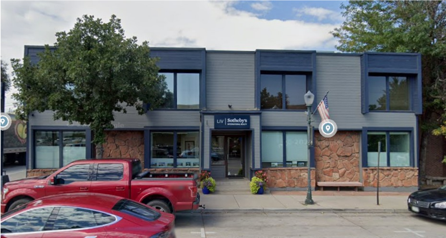
SUBJECT: EXTERIOR OF BUILDING
