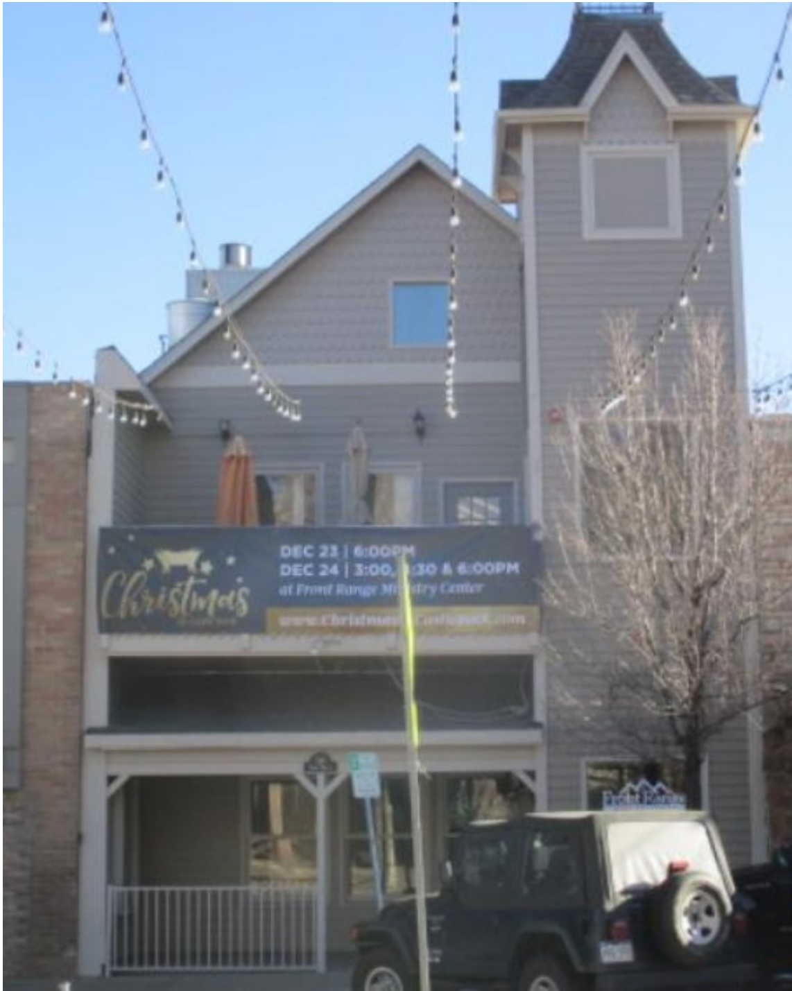
SUBJECT: EXTERIOR OF BUILDING
