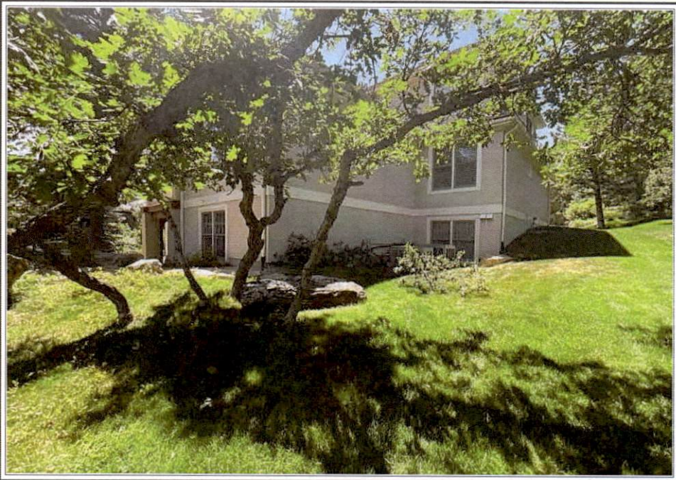
REAR OF SUBJECT PROPERTY
