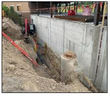
• WW Clyde Contracting is installing storm sewer pipe in Filing #4 of Canyons Subdivision (DV#2023-323).
