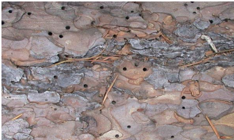
Figure 22 Ips beetle bore holes in pine.
