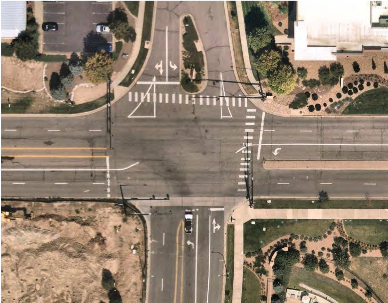
County Line Road and Erickson Boulevard
