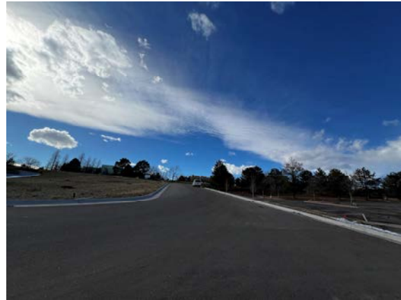
View of unnamed interior roadway towards Inverness Parkway, subject to the left
