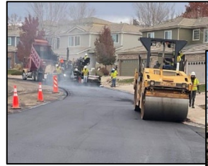
installing the top lift
