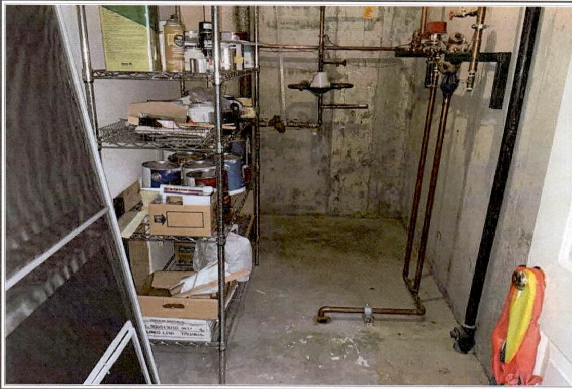
Basement Unfinished Area
