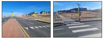
of an engineering analysis, additional street signage and pavement markings were recommended. Advance pedestrian warning signs and shark teeth yield pavement markings were implemented to increase visibility. After implementation, staff received a thank you from the resident.
