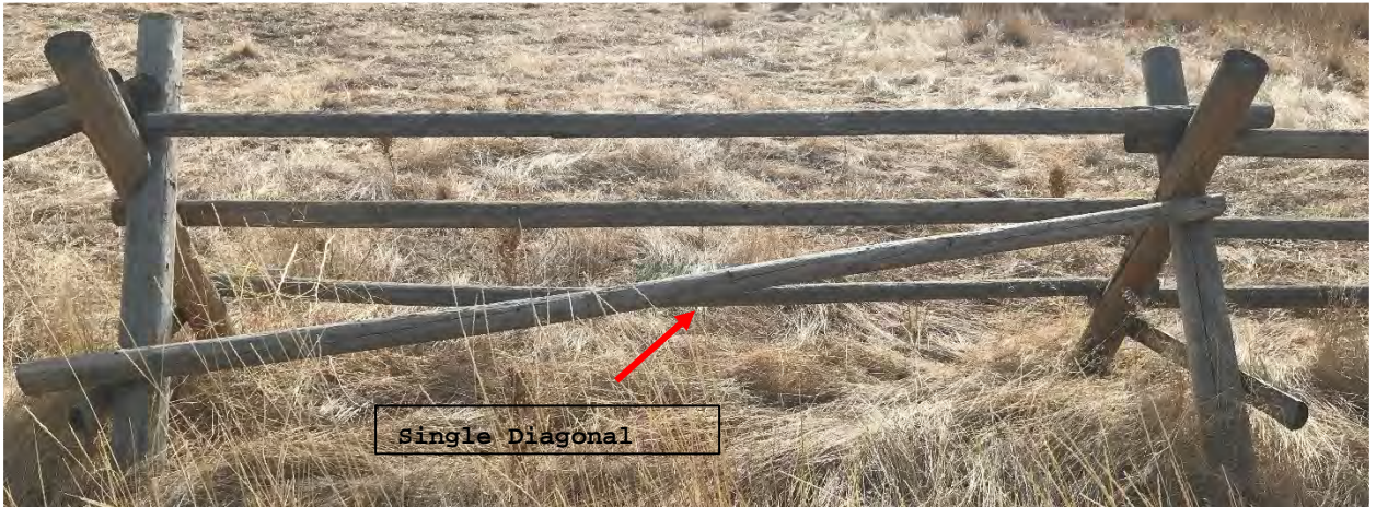
Figure 4. Buck and rail sections with a top pole secured and a diagonal brace pole.
