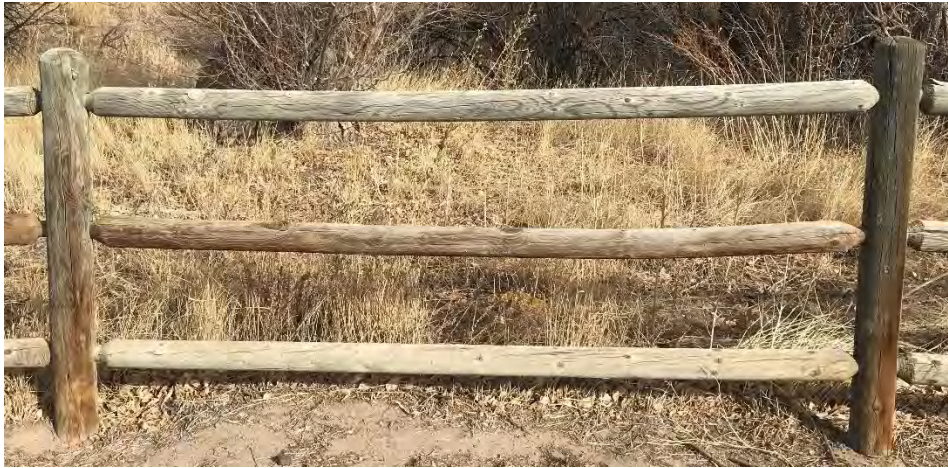
Figure 7. One complete section of post and rail fencing
