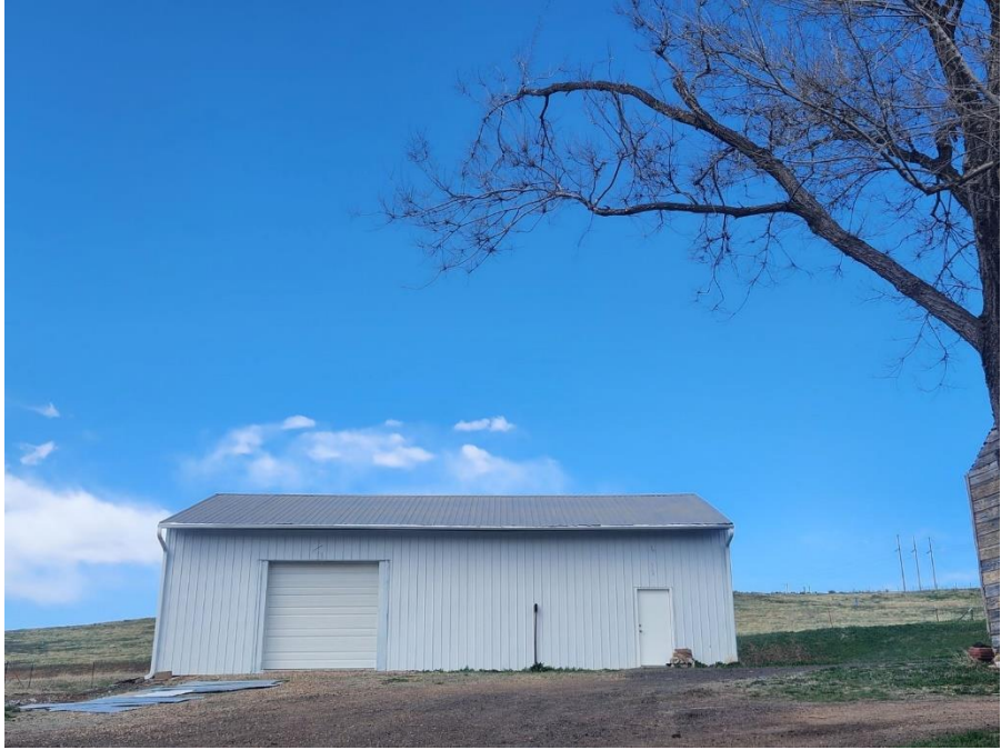
PHOTOGRAPH OF EXISTING SHED BUILDING
