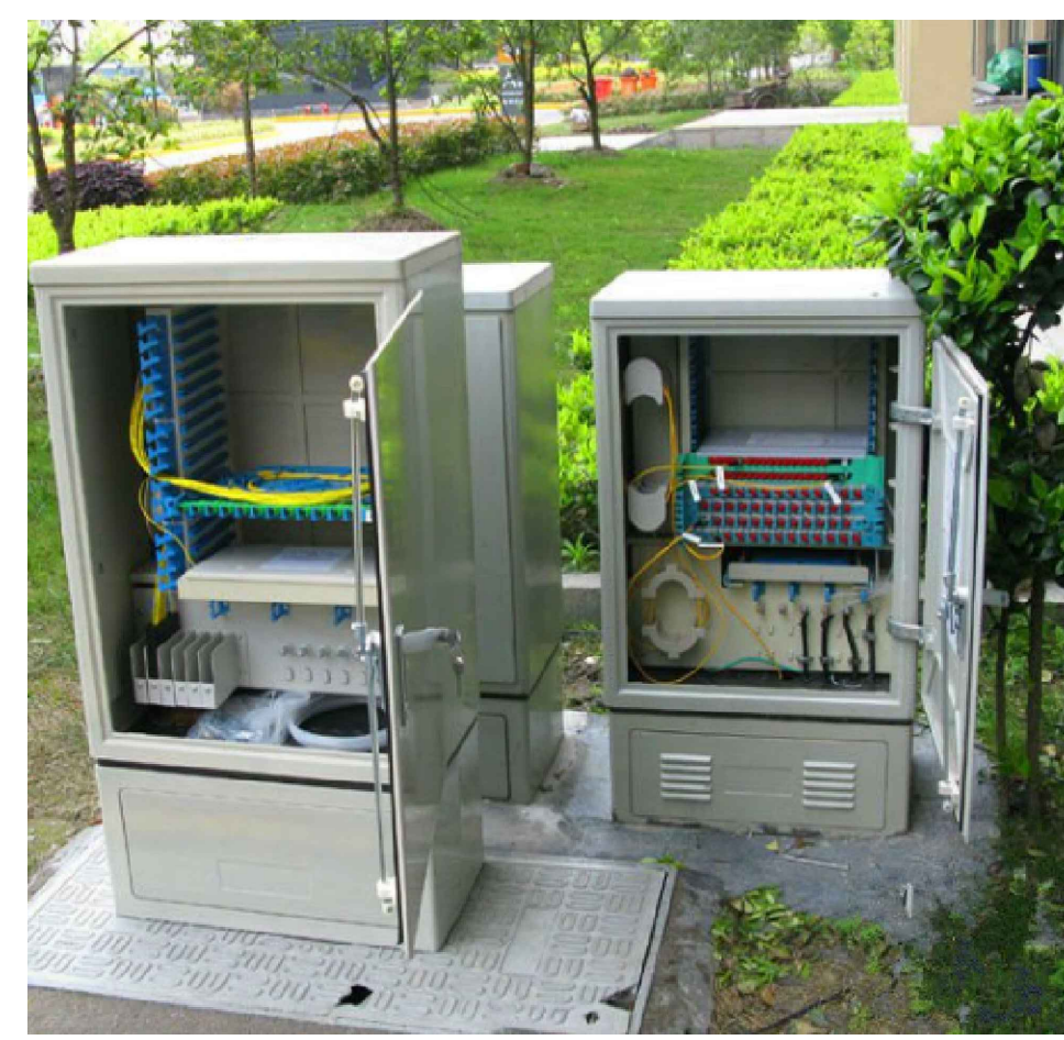
EXAMPLE COMMUNICATION CABINET N.T.S
