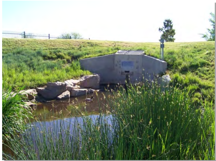
Photograph EDB-2. The initial surge volume of this EDB is contained within the boulders that surround the micropool.
