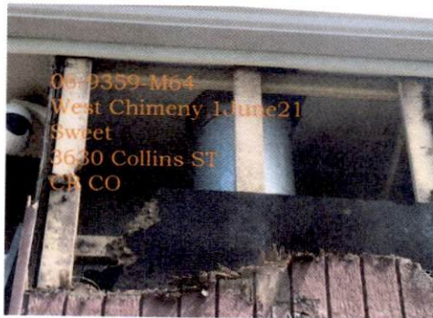
Image R0085016 Fireplace Abandoned 2010 Front Chimney Removed 2021 Hail Damaged Exterior remains un-repaired.
