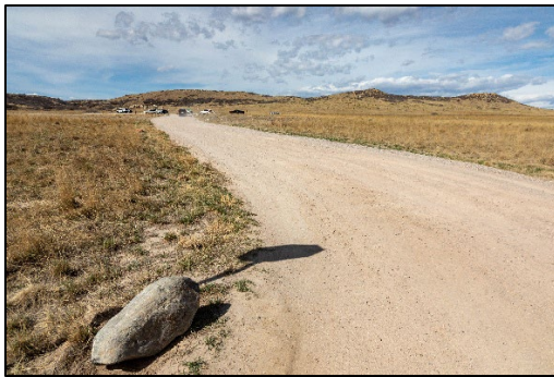
Before Dirt Driveway
